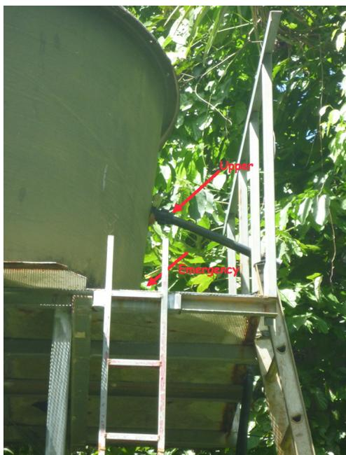
Safety arrangement – the water supply is taken from the middle of the tank (“Upper”). A second supply line (“Emergency”) is taken from the bottom – and has an easy to reach tap at ground level – if you have a serious water issue – you have lost only ½ your tank of water. Don't forget to turn the emergency valve off after it's all fixed!!
